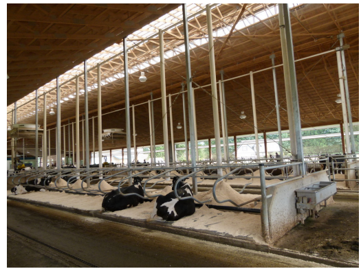
Figure 3 Automatic bedding delivery system
