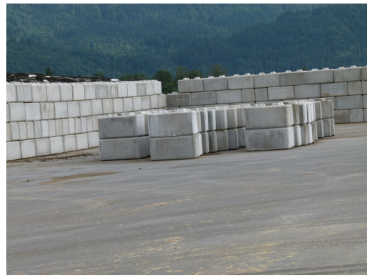
Figure 9 "Lego" concrete blocks for silo
