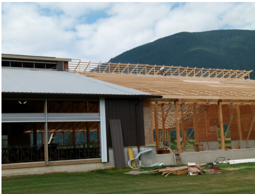
Figure 15 Over-shot ridge ventilation
