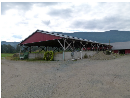
Figure 11 Roofed rectangular manure storage
