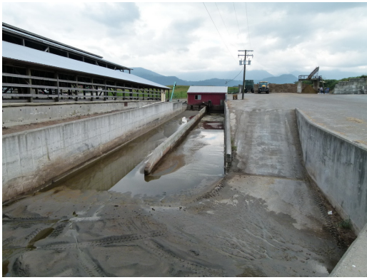
Figure 13 Sand settling lane
